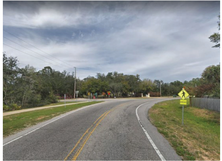
East Bay Boulevard in the Vicinity of Cedar Street - Note the poor condition of the center and edge lines
